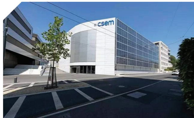
70 kWp BIPV system in Switzerland
